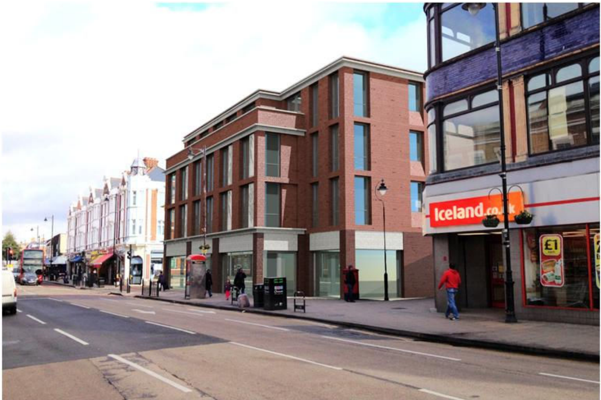
View north along High Road
